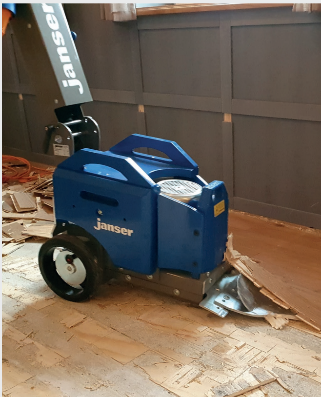
Operation with the parquet blade Dynamic shape suitable for removing all types of parquet floors. Solid parquet, two-layer and multi-layer parquet
